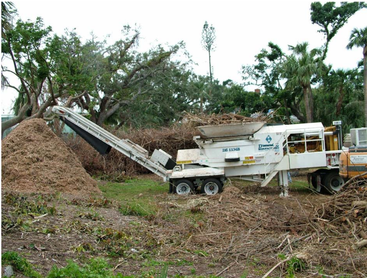
Figure 9. Mulching Brazilian pepper as part of exotic removal program.
