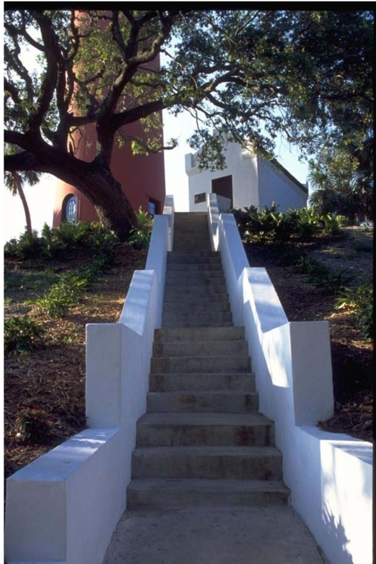
Figure 19. Looking up stairs to Jupiter Inlet Lighthouse and oil house.
